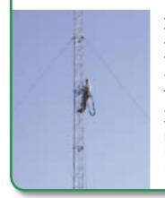
A wind generator tower is very often more expensive than the turbine. The tower puts the turbine up in the "fuel" the smooth strong winds that give the most energy. Wind turbines should be sited at least 30 feet (9 m) higher than anything within 500 feet (152 m).
